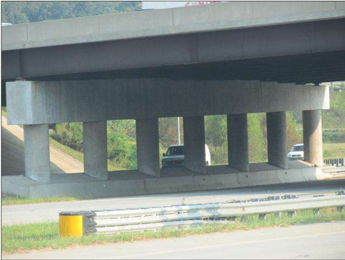
PIER 1 LOOKING SOUTH
