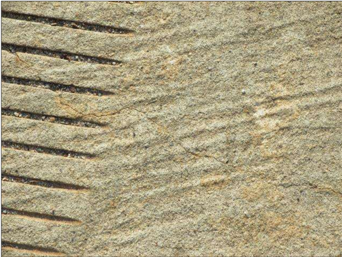
HL. TRANSVERSE CRACKS IN ALL SPANS
