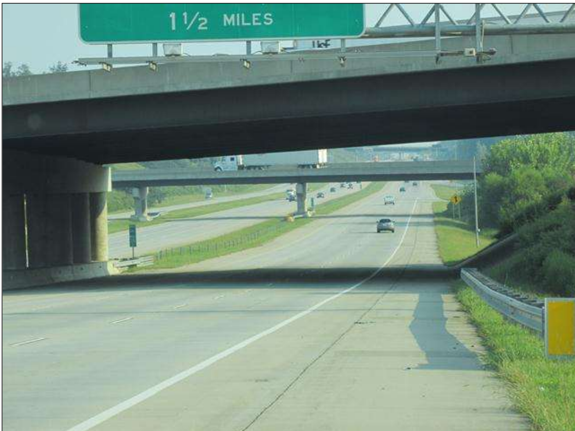
WEST OPENING, SPAN 3
