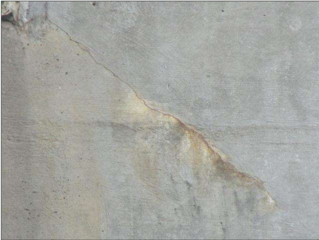
CRACKS IN BOTH ABUTMENT BACKWALLS
