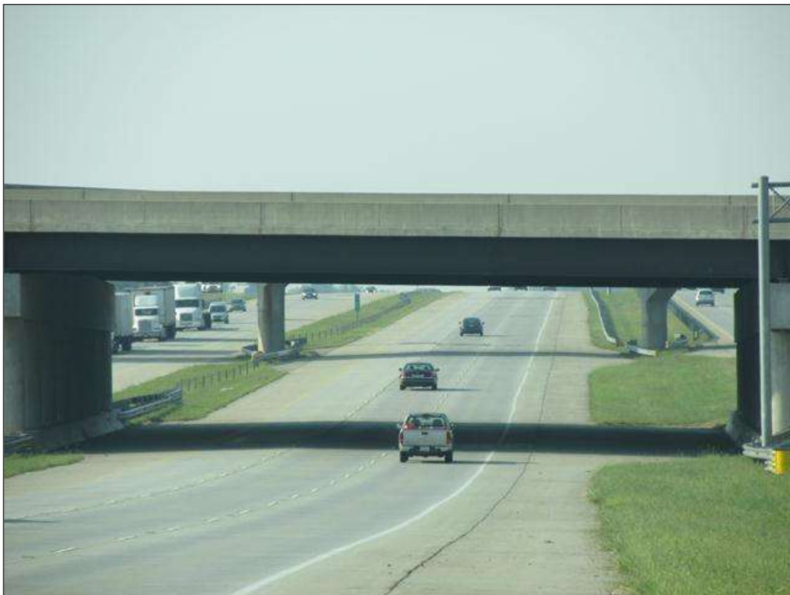
EAST OPEINING, SPAN 2
