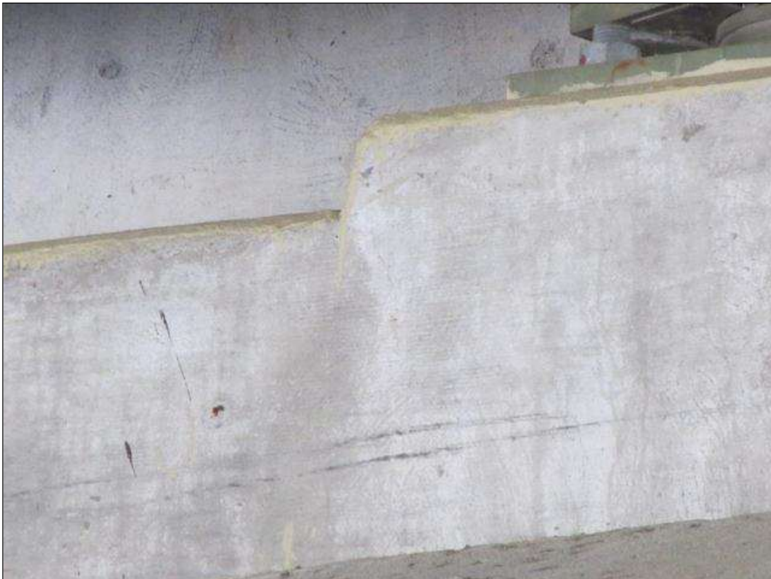
HL. CRACKS IN THE ABUT. CAP STEPUPS
