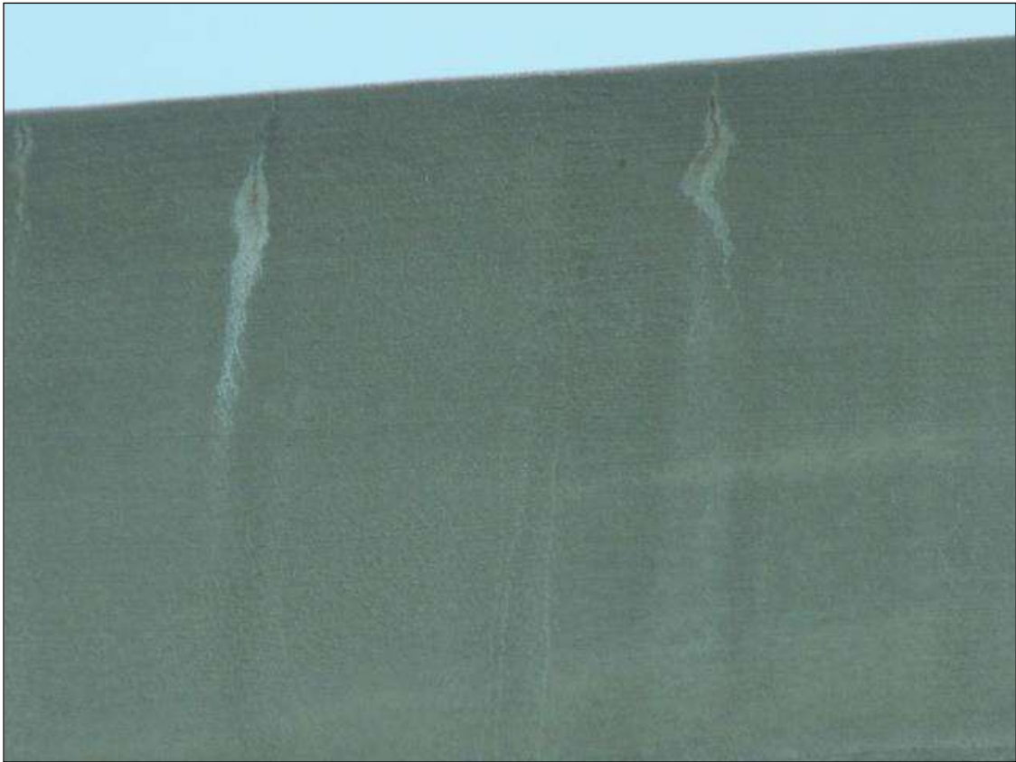
CRACKS IN BOTH RAILS
