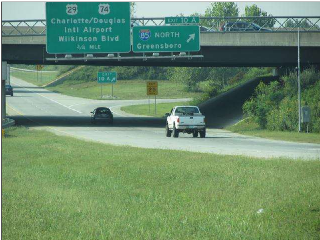
EAST OPEINING, SPAN 3
