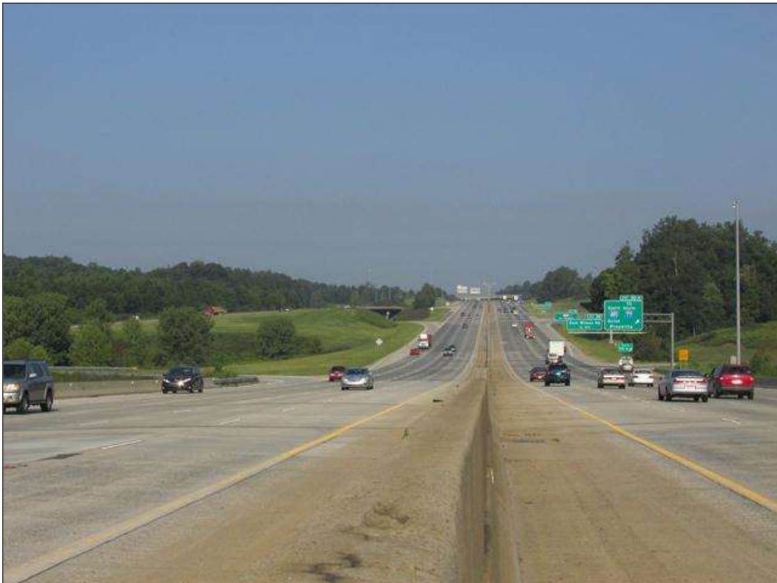
GUARD RAIL LOOKING SOUTH
