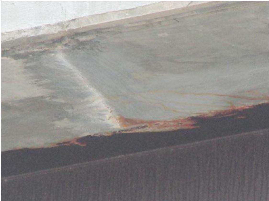
CRACKS IN BOTH OVERHANGS
