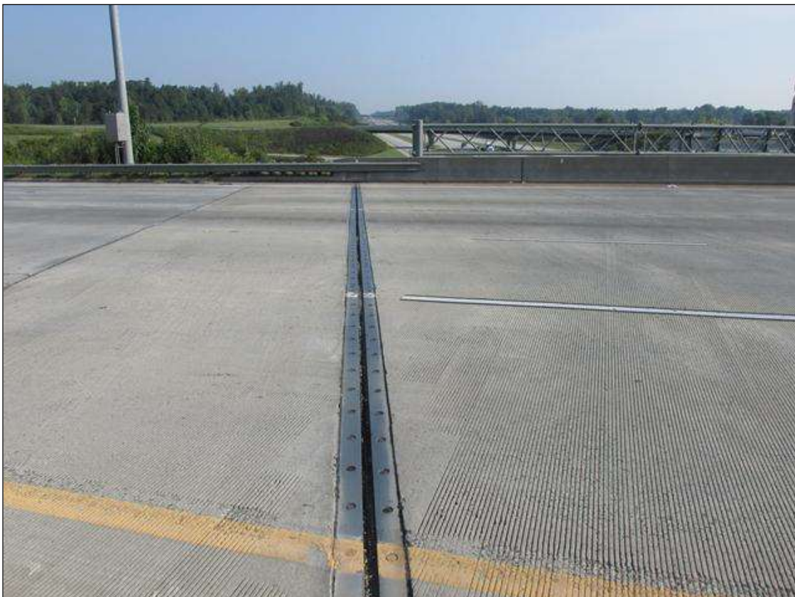
EXPANSION JOINTS AT BOTH ABUTMENTS
