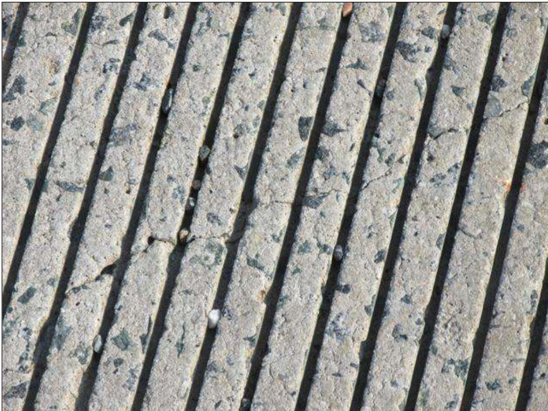
CRACKS IN THE SPAN ENDS
