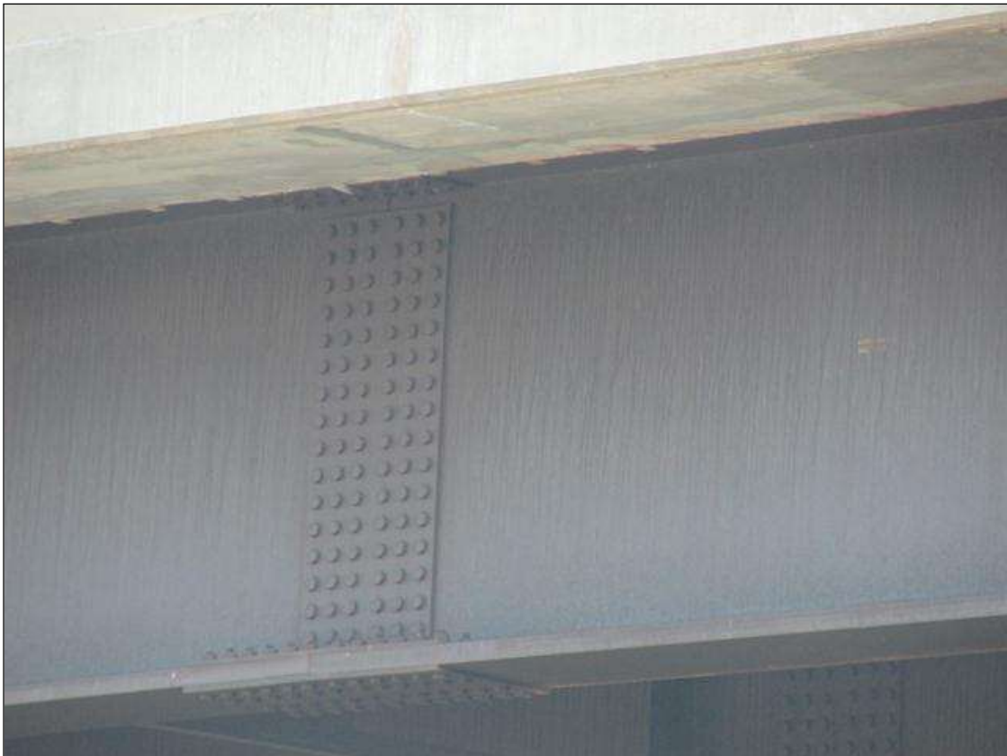
SPLICE PLATES IN ALL SPANS
